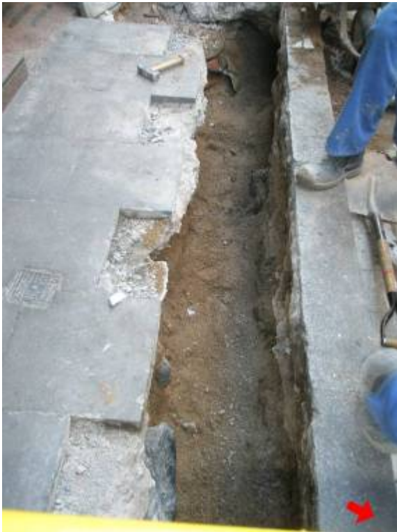
Tram final Rasa 100
